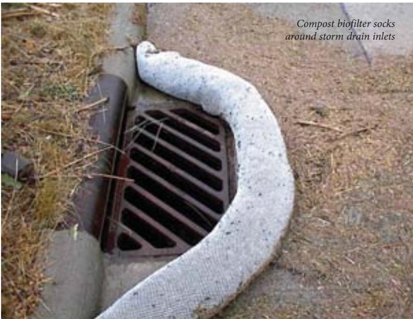
*Compost biofilter socks around storm drain inlets*
