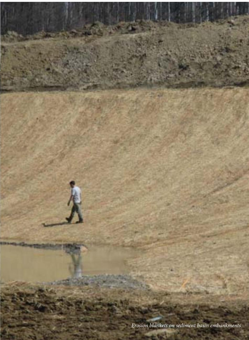
*Erosion blankets on sediment basin embankments*
