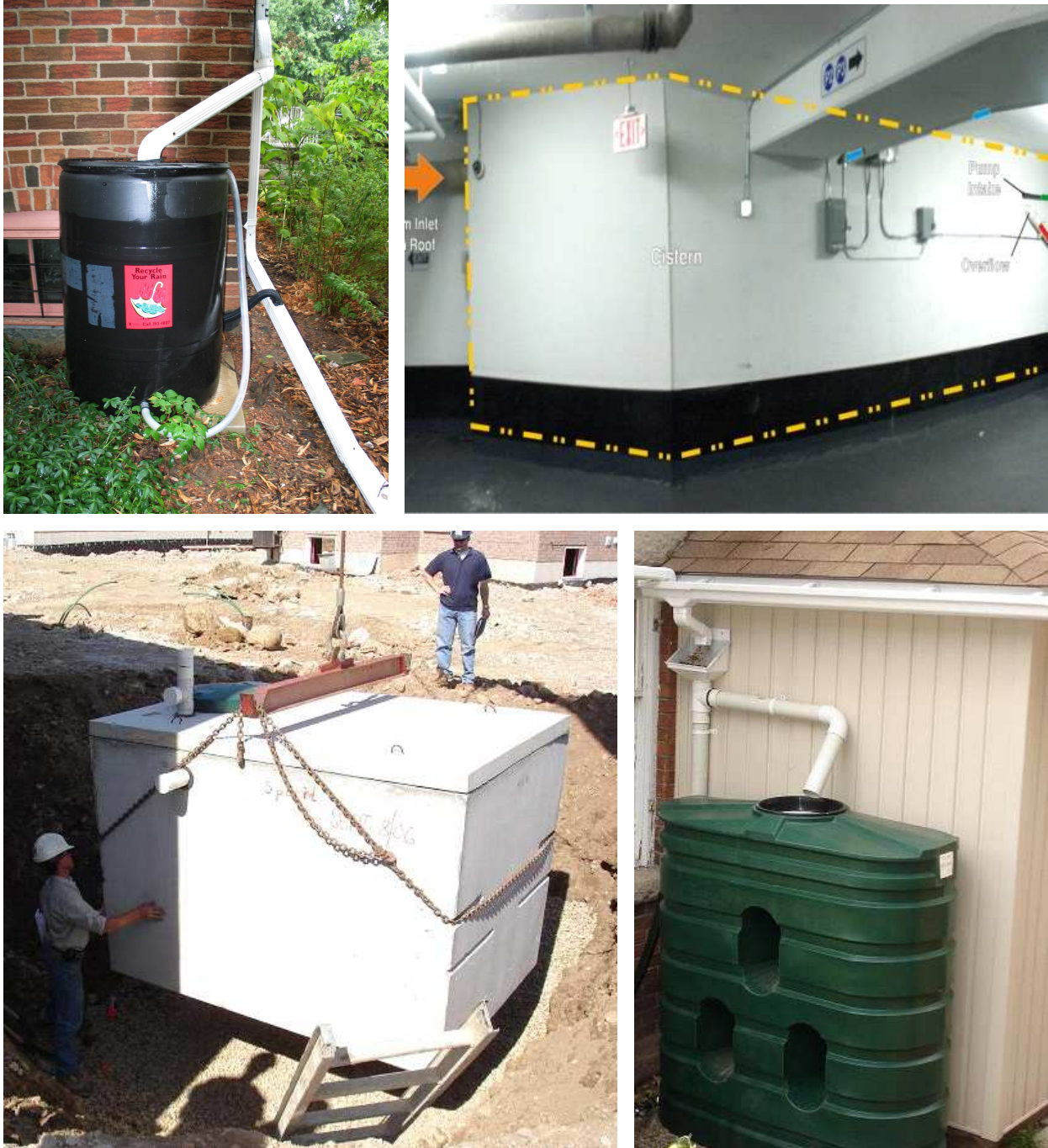
Clockwise from top left: typical plastic rain barrel; cast in place concrete cistern integrated within a parking garage (Source: TRCA); above-ground plastic cistern; underground pre-cast concrete cistern (Source: University of Guelph)
