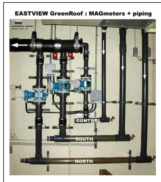
Figure 6 Piping and MAGmeter layout
