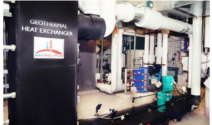
Figure 1. The geothermal heat exchanger in the basement mechanical room of the Earth Rangers Centre for Sustainable Technology.
