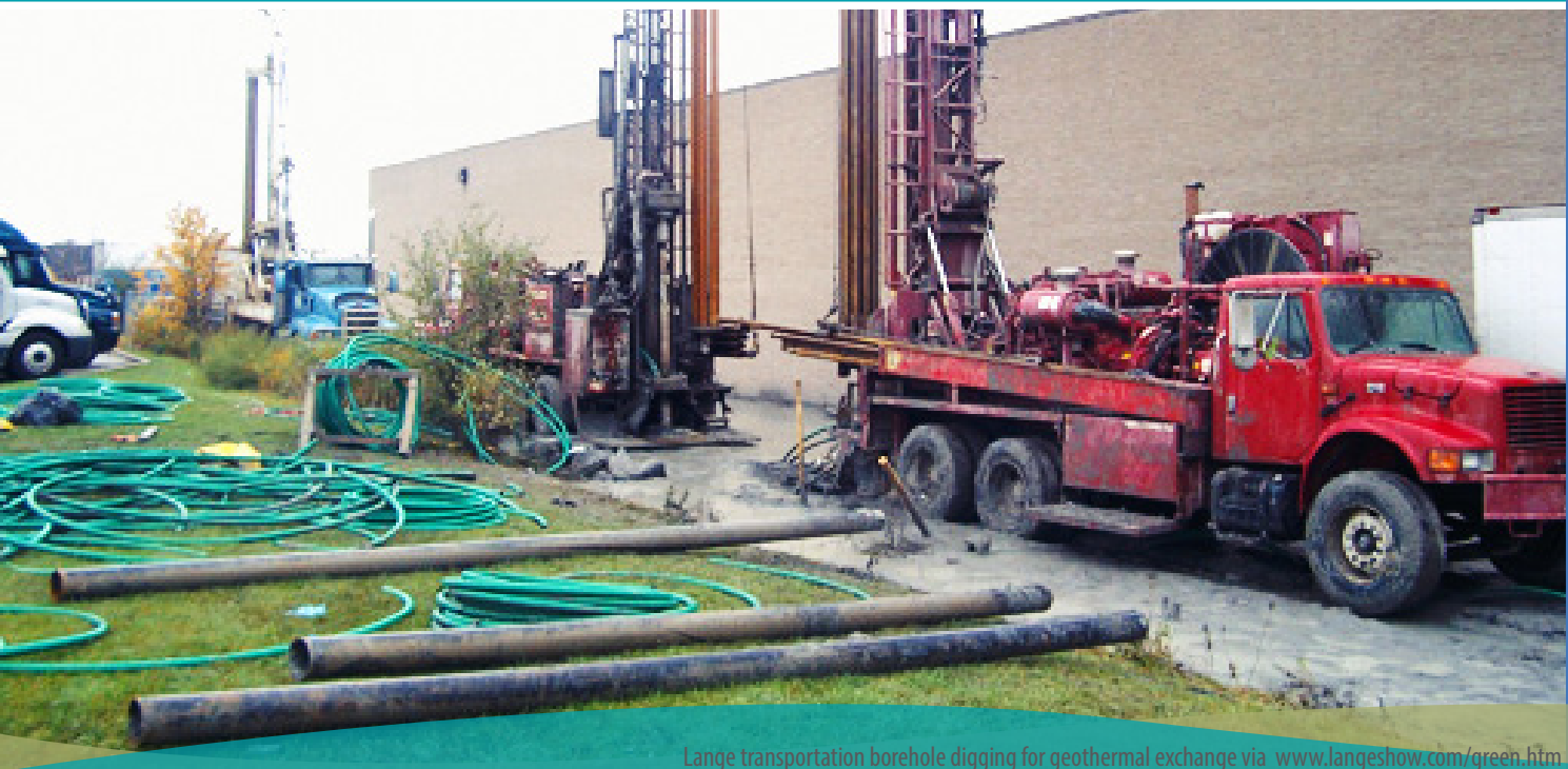
Lange transportation borehole digging for geothermal exchange via www.langeshow.com/green.htm
